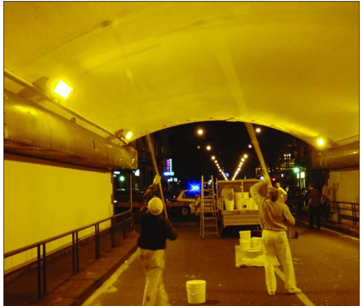
Photocatalytic paint is being tested in Europe to absorb smog.
